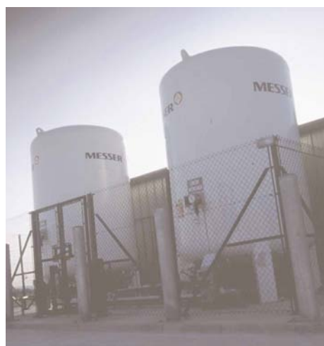
20,000L Liquid Nitrogen Dual Reservoir System
