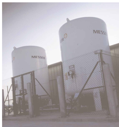
20,000L Liquid Nitrogen Dual Reservoir System
